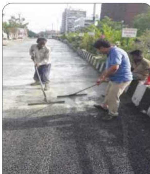
View of pouring of grout and squeezing on high voids bituminous mix
